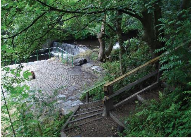
Looking down steps to weir area in 2006
